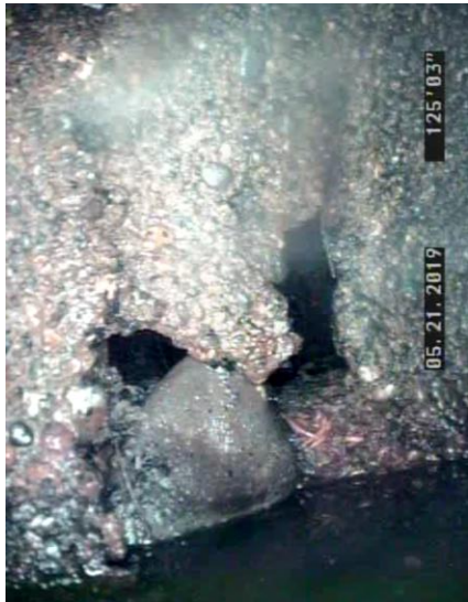
Broken Sides of Concrete Pipe Exposing Soil (125 ft.)
