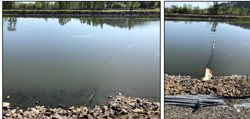
FIGURE 2.3.13 FACULTATIVE LAGOON BAFFLES
