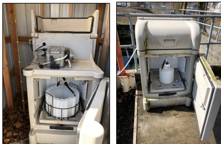
FIGURE 2.3.11 INFLUENT AND EFFLUENT SAMPLER
