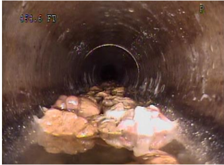
Apparent Flat Area near Cleanout (464.6 ft.)
